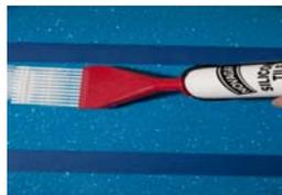
4. The adhesive cures quickly, so work with small runs so tiles can be placed within 2-3 minutes, to ensure the adhesive does not skin over before placement. Remove any excess squeeze-out from between and around tiles, and wipe off any adhesive from tile surface before it cures using paper towels and solvent.
