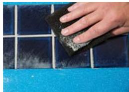
9. Continue smoothing the grout lines and **COMPLETELY** cleaning off all excess grout and haze from the tile surfaces, as it is extremely difficult to remove after the silicone grout cures. Rinse soapy residue. A final gentle wipe with paper towel and solvent may help.
