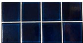
10. Allow 24-78 hours before placing into service. Working times and cure times are very dependent on humidity and temperature.
