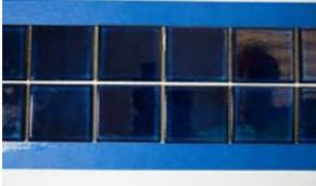
7. Again working in short runs (that can be finished within 10-15 minutes), apply Novagard silicone grout to the grout lines and use a smooth rubber float to press the grout completely into the tile joints.
